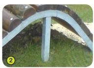
2- The frames are made of galvanised steel.
