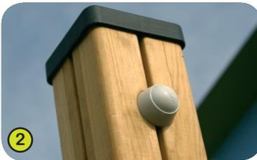
2- **The vertical 95mm square post** are made of laminated timber, which have not been treated with chrome or arsenic. Splinter-free, the laminate provides great strength and dimensional stability. The posts are protected from wear and tear caused by fungi, insects and termites.
