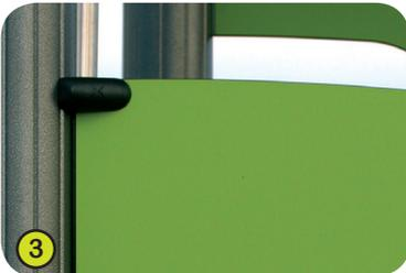
3- **The play walls and roofs** are coloured panels made from a compact material 13mm thick, 70% softwood fibre and 30% thermosetting resin, which stands up to weathering very well.
