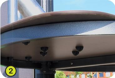
2- **The platforms** are made from a 12.5mm thick, textured, non-slip compact material (HPL).
